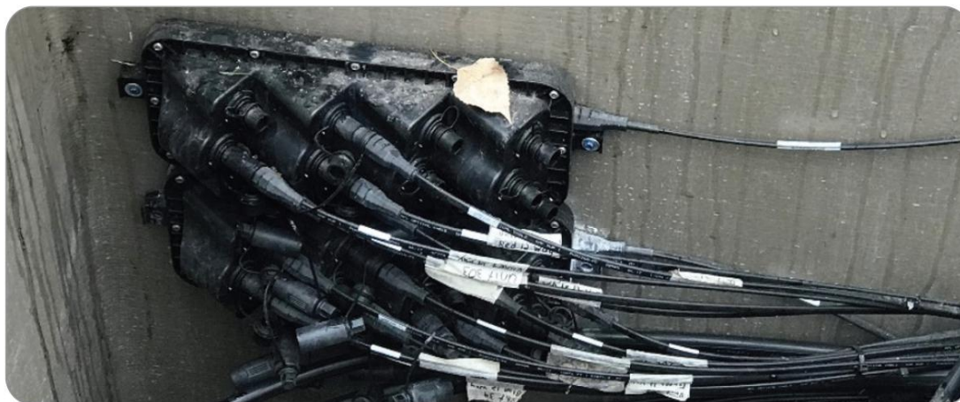
Figure 4 — Handhole Mount Application
